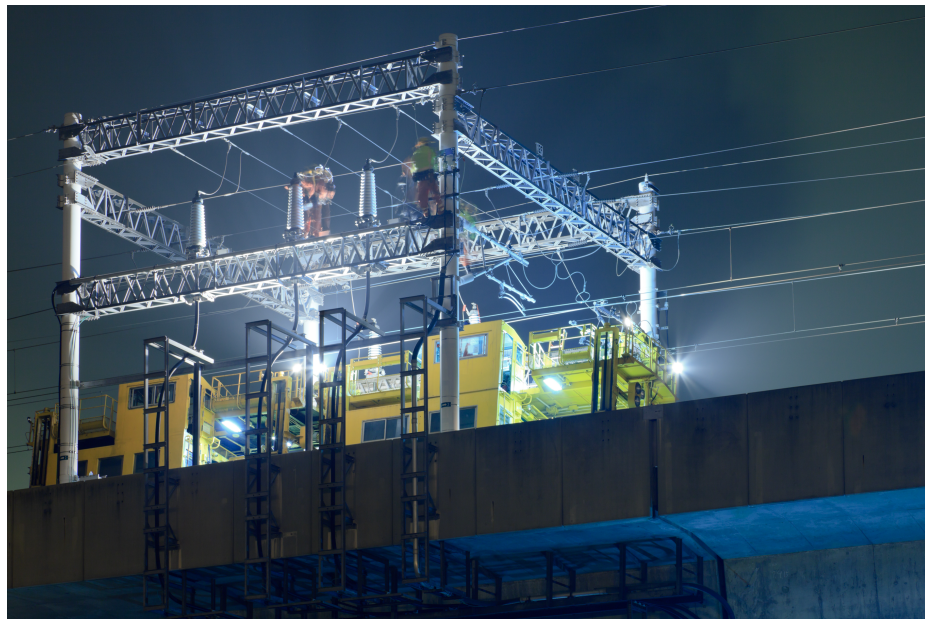
Fig14: Railway maintenance team working overnight to keep the trains running
