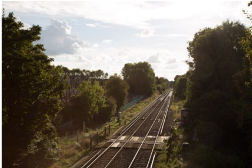
Fig2: Third rail supply to trains (broken at crossing point to prevent electrocution)
