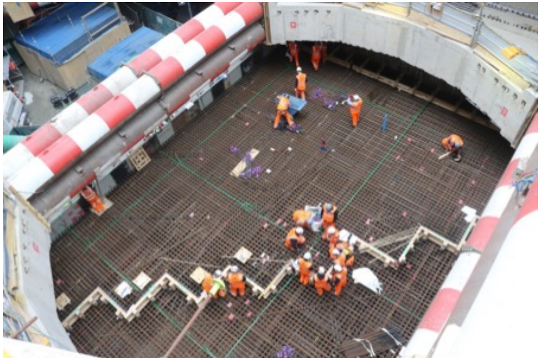
Fig7: Crossrail station earth mat under construction (Jonathan King FIET, 2018)
